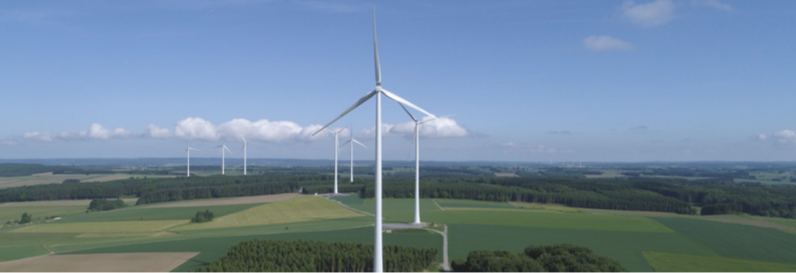
/ Wind farm – Wincrange /
